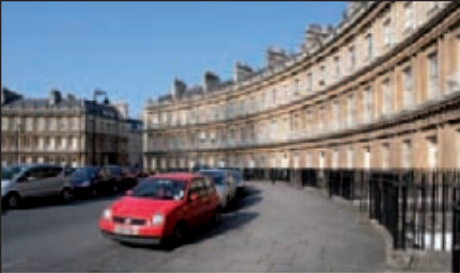
Above left The Circus, an elegant 18th-century terrace designed by John Wood, Bath
