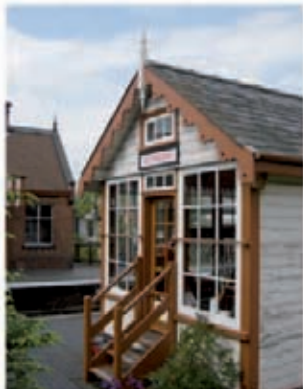
Above Little station on the North Norfolk Railway Poppy Line, Weybourne
