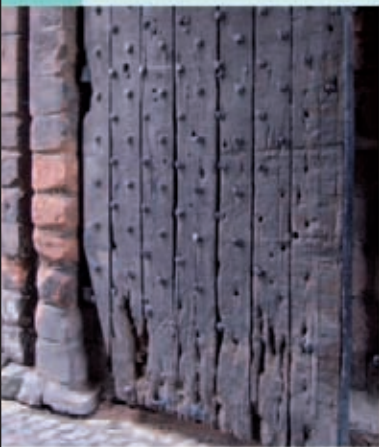
Above Ancient wooden door at Carlisle's 12th–14th-century castle
