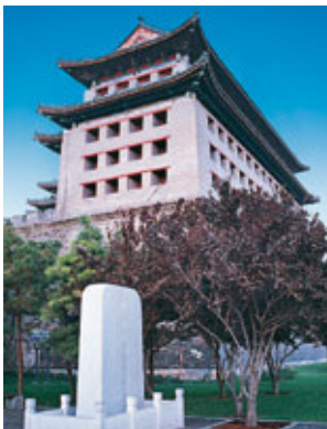
Southeast Corner Watchtower
