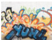
Graffiti-daubed wall in the factory compound
