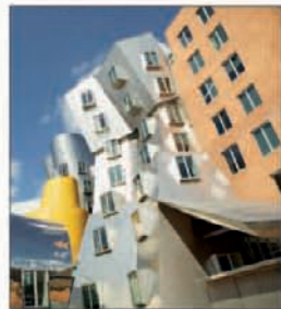
The Stata Center designed by Frank Gehry ⑨
