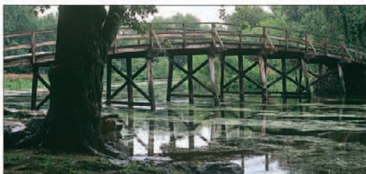
North Bridge in Minute Man National Historical Park
