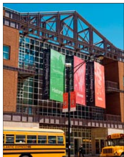
Front of the newly renovated Chicago History Museum ①
