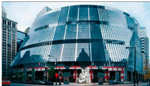
The massive James R. Thompson Center, Standing Beast in foreground
