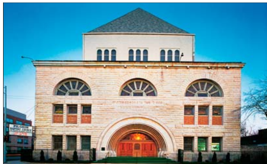
Façade of the Pilgrim Baptist Church, with its distinctive doorway
