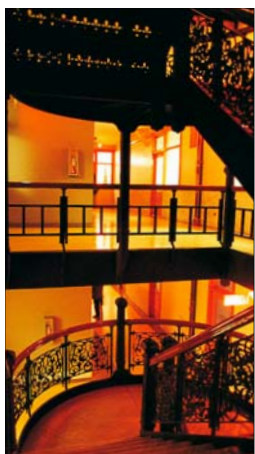
The Monadnock Building's fireproof wrought-iron staircase
