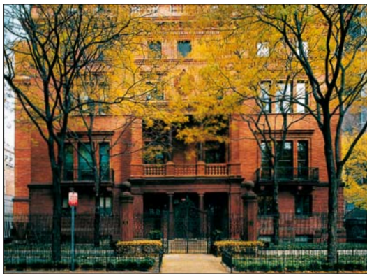
Façade of 1500 North Astor Street, with its Classical detailing
