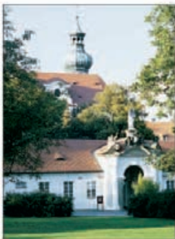
Břevnov monastery, designed largely by the Dientzenhofers
