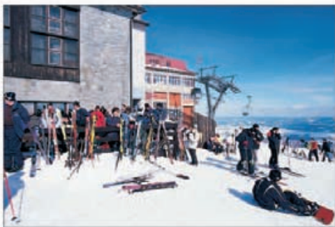
Chairlift station in Skalnáté pleso, the High Tatras
