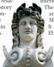
Detail above Karlovy Vary Theatre entrance
