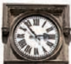
Clock on Old Town Hall Tower
