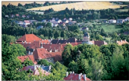
View of the monastery buildings in Plasy
