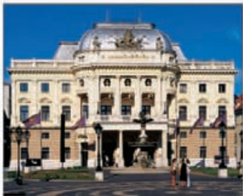
The Slovak National Theatre in Bratislava (see p282) was built in Neo-Renaissance style during 1885–8 by Viennese architects Ferdinand Fellner and Hermann Helmer , who specialized in designing theatres and opera houses.
