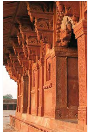
Entrance to Birbal's House
