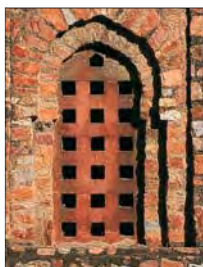
Detail of an arched window with jaali
