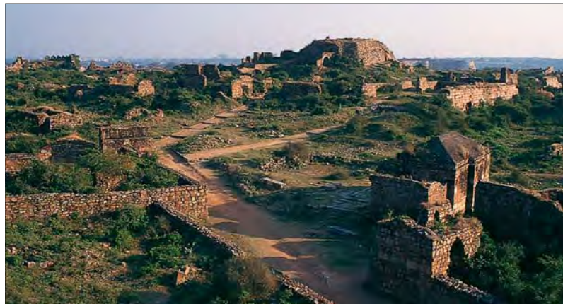
The crumbling ramparts of Tughlaqabad Fort
