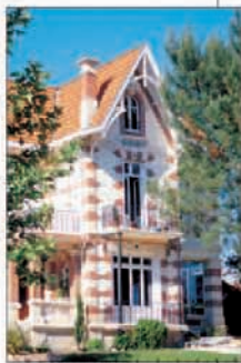
A villa at Arcachon
