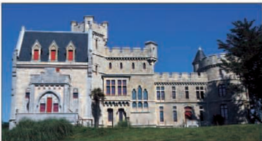
The sturdily built Neo-Gothic Château d'Abbadia at Hendaye
