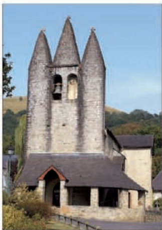
Bell tower with three steeples on the 16th-century church at Gotein, near Mauléon
