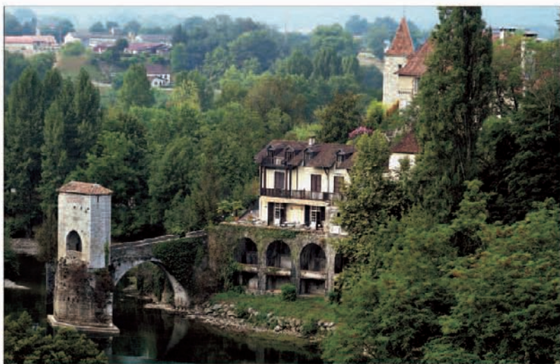
Pont de la Légende over the Gave d'Oloron at Sauveterre-de-Béarn, on an ancient route to Navarre
