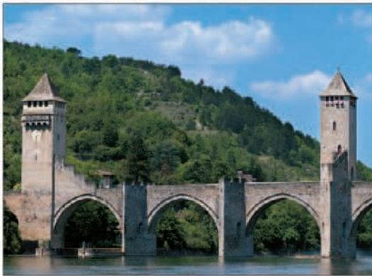
Pont Valentré, one of the most beautiful medieval bridges in Europe
