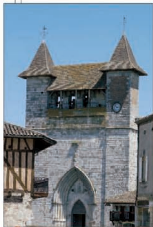
The fortified church at Villeréal
