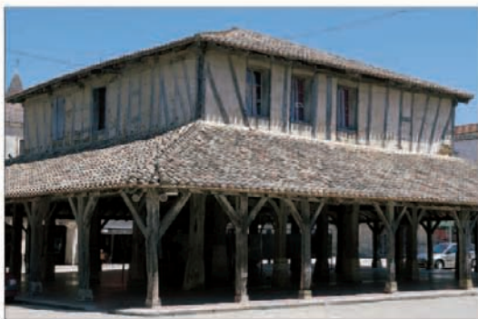
The late 14th-century covered market at Villeréal
