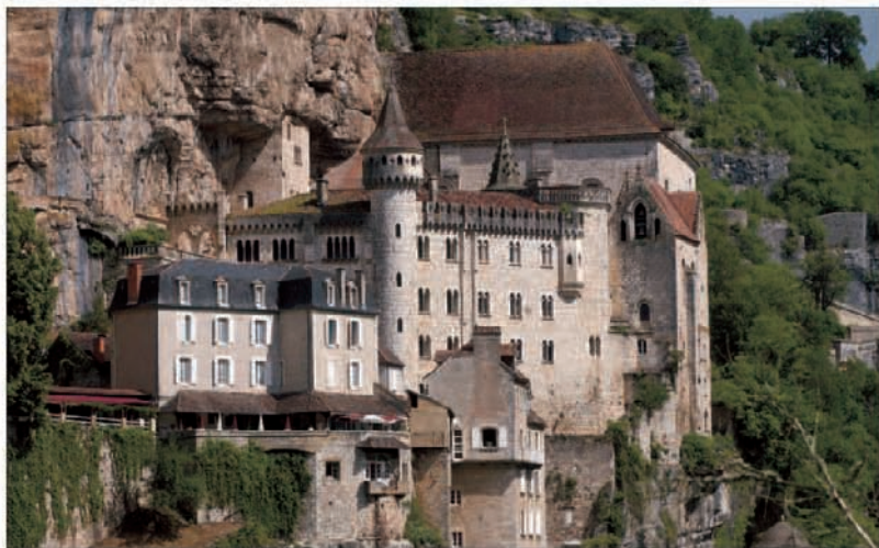
The crypt of St Amadour, built into the rock face
