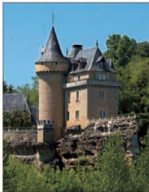
Château de Blecayre, between Thonac and Sergeac
