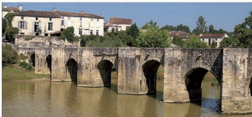
The ten-span Romanesque bridge at Barbaste
