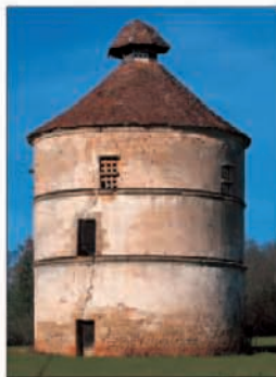
16th-century dovecote built by Galiot, lord of the manor of Assier
