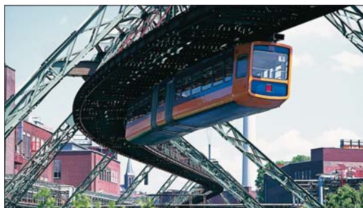
The unusual monorail, linking Wuppertal's six constituent towns
