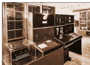
1941 Konrad Zuse constructs the Z3 calculator – the first digital "computer"
