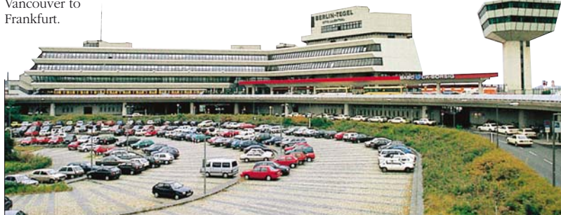
Car park and airport building at Tegel airport, Berlin
