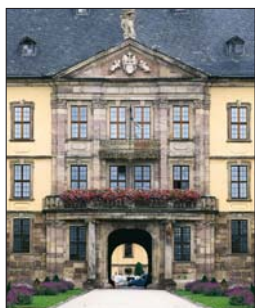
Projecting gate of the Baroque Stadtschloss in Fulda
