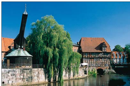
Eighteenth-century wooden crane in Lüneburg
