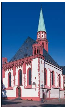
The early-Gothic Alte Nikolaikirche , in Frankfurt's Römerberg
