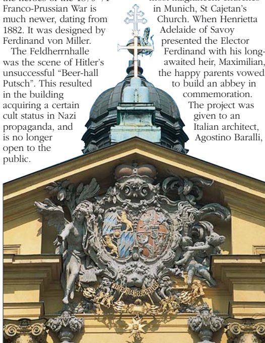
Pediment on the gable of Theatinerkirche, with copper dome behind
