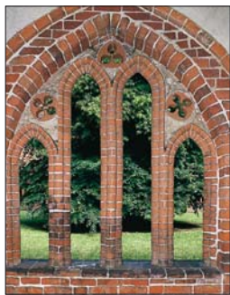
Gothic traceries of the cloisters in the Dom, Havelberg
