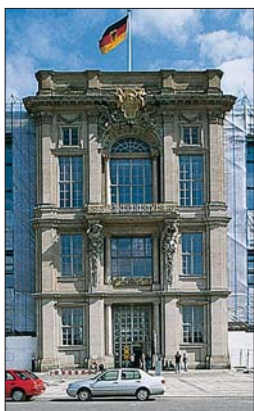
The surviving Stadtschloss portal fronting a government building
