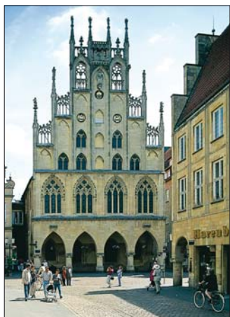
The beautifully restored façade of the late-Gothic Rathaus
