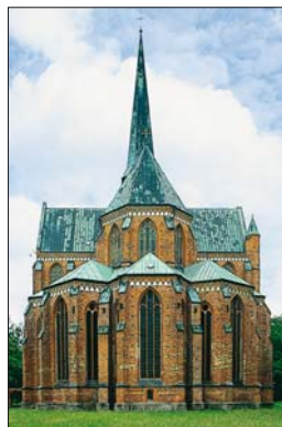
The monumental Cistercian Münster in Bad Doberan
