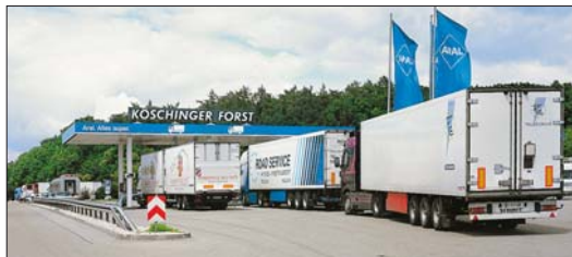
Petrol station at a motorway service area
