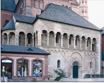
The front elevation of the St Gotthard-Kapelle in Mainz has upper galleries with arcades decorated with friezes – a common feature of Romanesque architecture.
