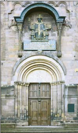
The northern portal of the Dom in Worms is framed by an offset architrave and flanked by pairs of columns, as are the portals of many other Romanesque cathedrals.
