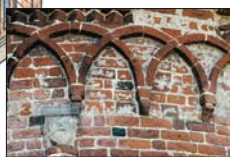
Friezes on the arcades , such as this interlaced motif made from brick, are frequently used as a decorative element, even in village churches.
