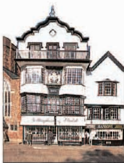
The timber-framed Mol's Coffee House (1596), Cathedral Close
