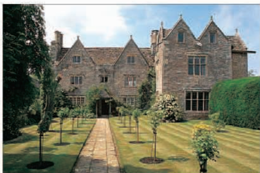
The formal entrance of the Elizabethan Kelmscott Manor
