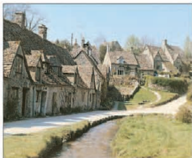
Arlington Row Cottages in Bibury, a typical Cotswold village, were built in the 17th century for weavers whose looms were set up in the attics.
