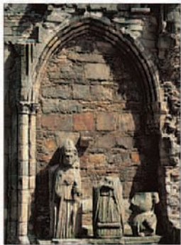
Details of the central tower of Elgin Cathedral
