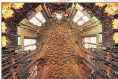
Rib-vaulting in the Thistle Chapel, St Giles Cathedral
