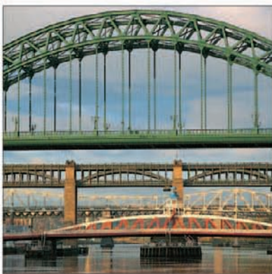
Bridges crossing the Tyne at Newcastle
