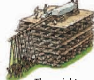
The weight of the lintel was supported by a timber platform.
