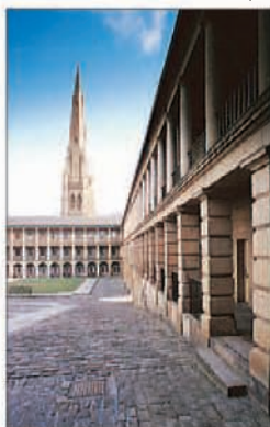
Halifax's Piece Hall (see p413), restored in 1976, is the most impressive surviving example of industrial architecture in northern England. It is the only complete 18th-century cloth market building in Yorkshire. Merchants sold measures of cloth known as "pieces" from rooms lining the cloisters inside.
