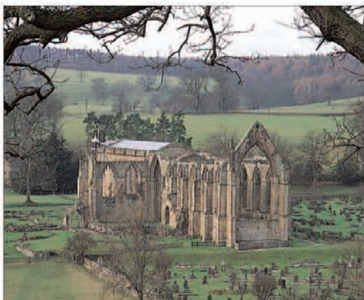
Extensive ruins of Bolton Priory, dating from 1154
