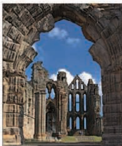
Medieval arches above the nave of Whitby Abbey
