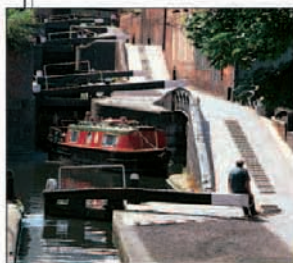
The Farmer's Bridge is a flight of 13 locks in Birmingham. Locks are used to raise or lower boats from one level of the canal to another. The steeper the gradient, the more locks are needed.
