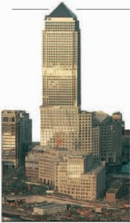
1991 Then Britain's tallest building, Canada Tower ( see p125 ), was erected as part of the huge Docklands development – London's financial centre
