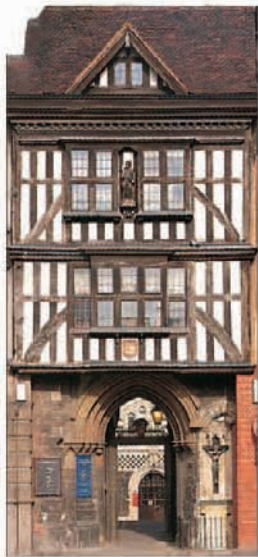
St Bartholomew's gatehouse
