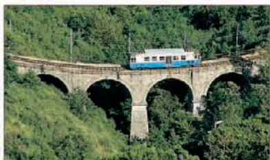
The Casella train crossing a viaduct
