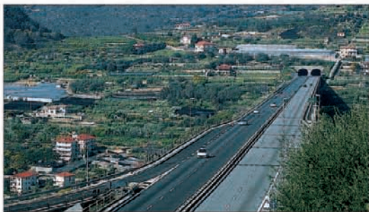
A stretch of the motorway linking Liguria's main towns
