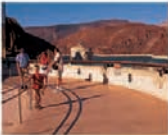
The top of the dam
