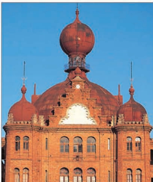
Neo-Moorish façade of the bullring in Campo Pequeno
