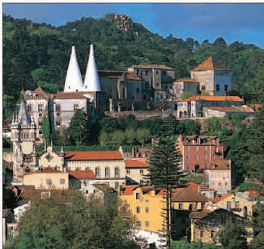
Chimneys of the Palácio Nacional de Sintra above the old town
