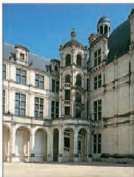
**The lantern tower, 32 m (105 ft) high, is supported by flying buttresses.**
