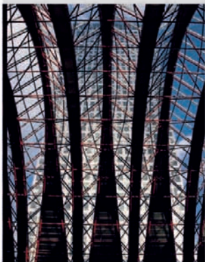
Vaulted glass roof, Canary Wharf DLR station
