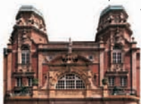
Restored façade of Richmond Theatre
