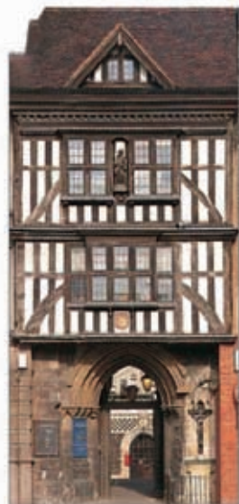
St. Bartholomew's gatehouse
