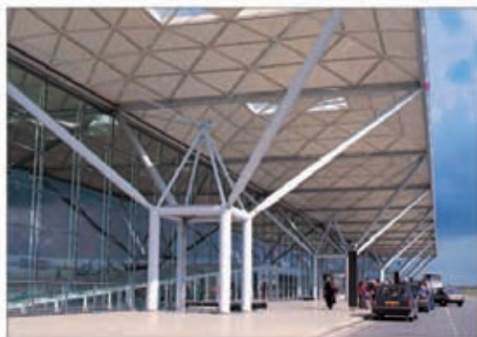
Entrance to Stansted's spacious modern passenger terminal
