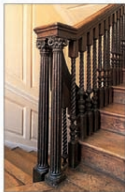
Burgh House staircase
