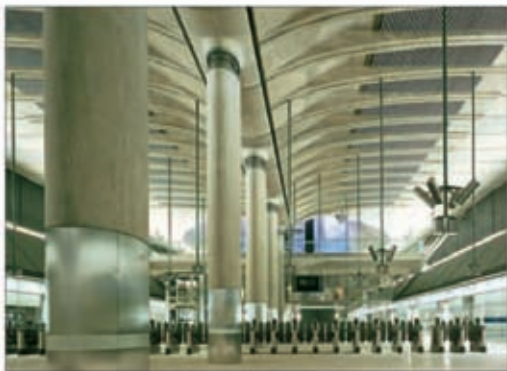
Concourse at Canary Wharf Station, Jubilee Line
