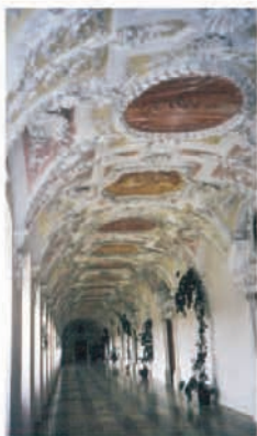
Stuccoed ceiling, Kloster Wessobrunn
