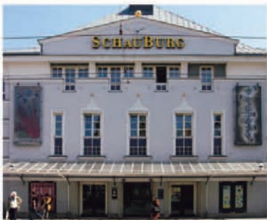
Exterior of Schauburg
