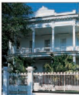
The second-floor galleries at Robinson House
