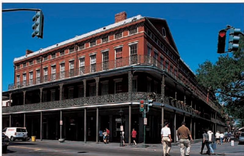
The Pontalba Buildings, the upriver side of Jackson Square
