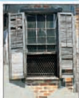
Brick, stucco, and timber walls
