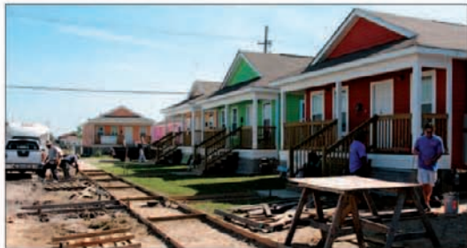
Homes being built in the New Orleans Musicians' Village
