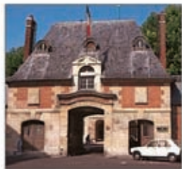
Entrance to Hôpital St-Louis ⑭
