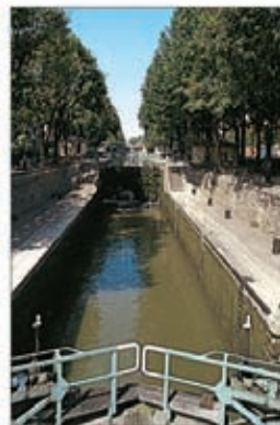
View from Rue E Varlin bridge ⑦
