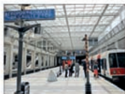
Charles de Gaulle airport RER station
