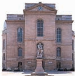
The facade of the Observatoire
