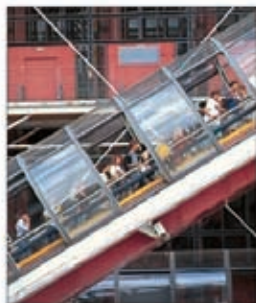
Escalators at the Pompidou Centre
