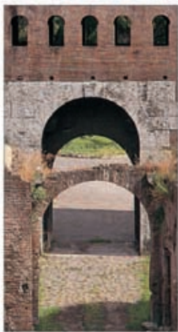
Porta Asinaria from inside the wall
