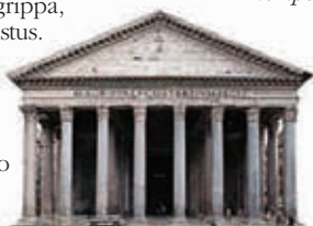
The portico, enclosed by granite columns
