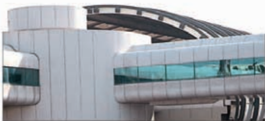
Part of the extension to Fiumicino airport
