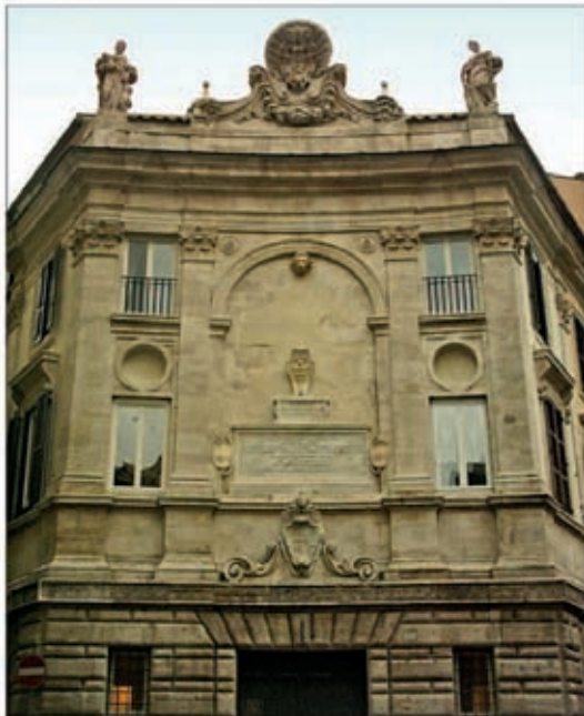
Facade of the Banco di Santo Spirito, built to resemble a Roman arch
