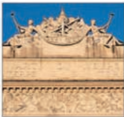
Detail of facade, Teatro Argentina
