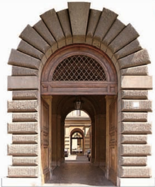
Rusticated doorway of the Palazzo dei Convertendi
