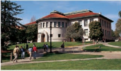
Wellman Hall, University of California, Berkeley
