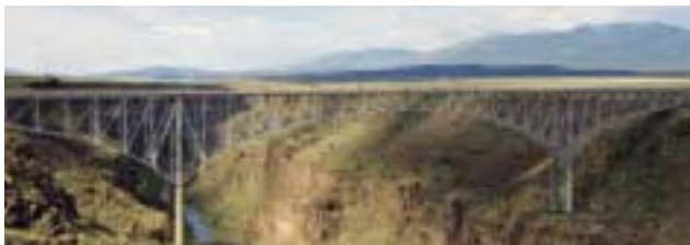
A spectacular view of the Rio Grande Gorge Bridge
