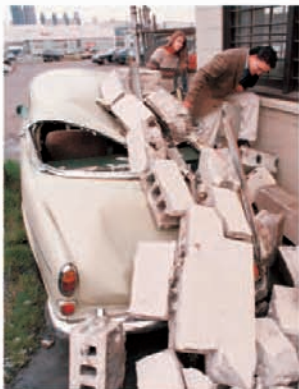
Devastation after the 2001 earthquake
