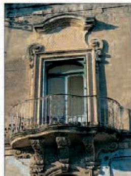
A Baroque balcony in the centre of Palazzolo Acreide
