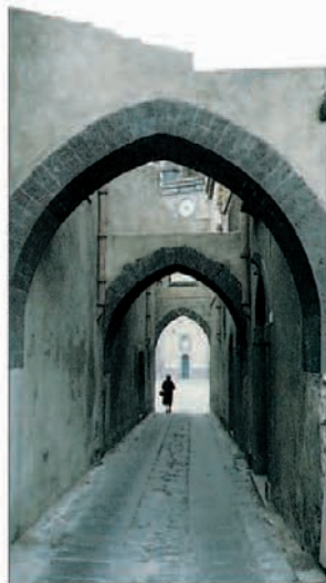
The restored Via degli Archi with its cobbled lava paving
