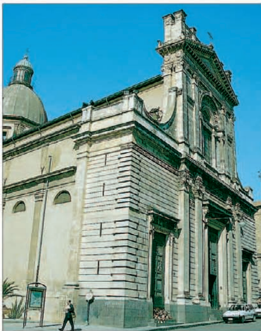
San Giuliano, displaying some 20th-century architectural features
