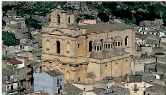
Santa Maria la Nova, at Scicli, rebuilt in the Neo-Classical style
