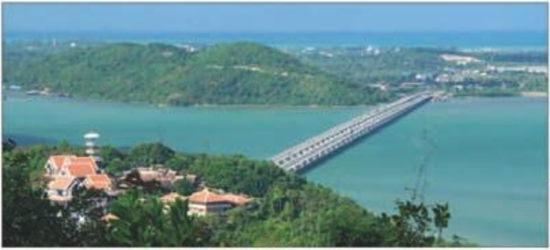
Thailand's longest concrete bridge connecting the mainland to Ko Yo
