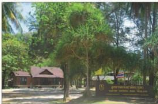
Bungalow housing the Ko Tarutao park headquarters, Ao Pante Malaka
