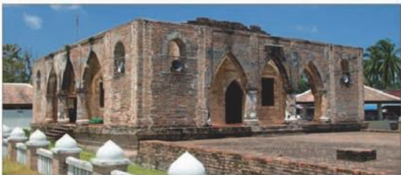
The partially built structure of the 16th-century Kru Se mosque, Pattani
