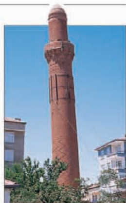
The Eğri (Leaning) Minaret, built by the Seljuks in the 13th century
