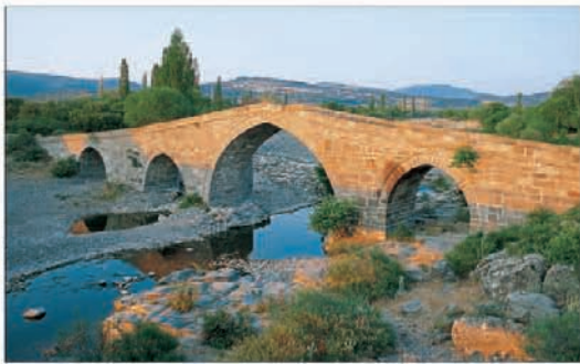
Humpbacked Ottoman bridge on the outskirts of Behram Kale
