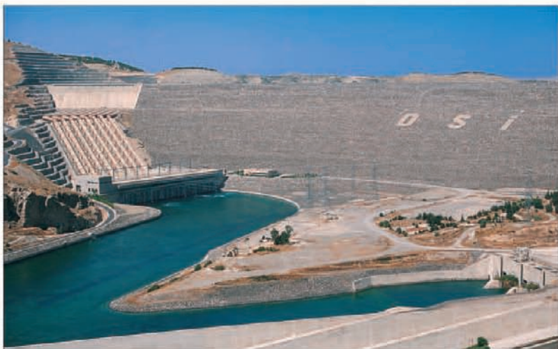
The Atatürk Dam, centrepiece of the GAP (Southeast Anatolian Project)
