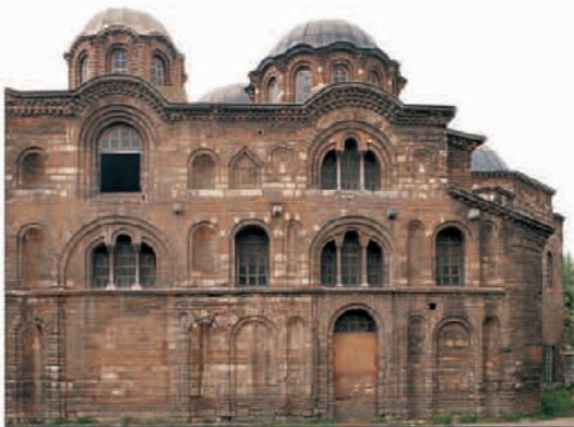
Byzantine façade of the Church of the Pammakaristos
