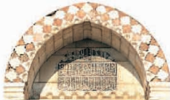
Entrance arch, Mosque of the Three Balconies
