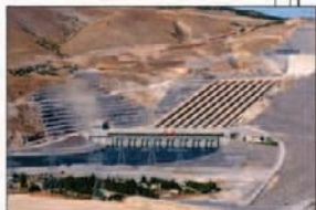
The massive Atatürk Dam
