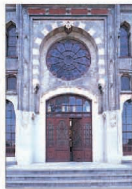
Sirkeci Station, final destination of the historic Orient Express
