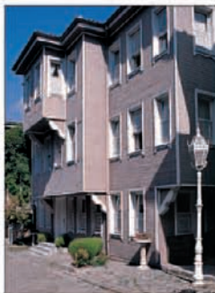
Restored Ottoman house on Soğukçeşme Sokağı
