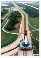
The Crawlerway is a double pathway, 180 ft (55 m) wide. It has been specially designed to withstand the weight of the shuttle as it is taken to the launch pad by gigantic crawlers. The rock surface overlies a layer of asphalt and a 7-ft (2-m) bed of crushed stone.
