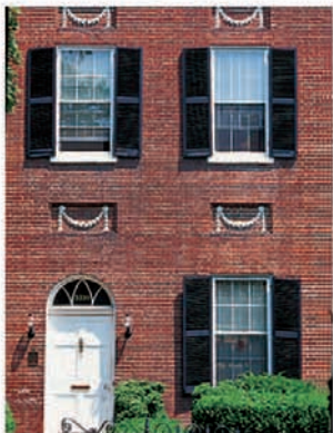
N Street house
