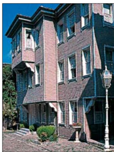
Restored Ottoman house on Soğukçeşme Sokağı
