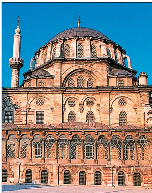
The Baroque Tulip Mosque, housing a marketplace in its basement
