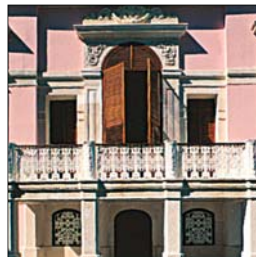
Façade of Çadır Pavilion, which has now been refurbished as a café
