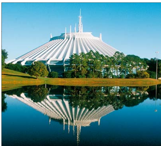
The futuristic building that houses the Space Mountain® ride
