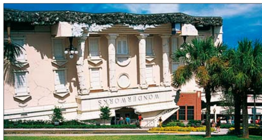
The upside down façade of WonderWorks
