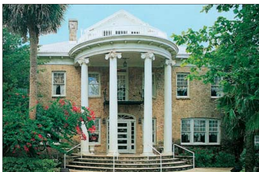
The grand Porcher House, on the edge of Cocoa's leafy historic district
