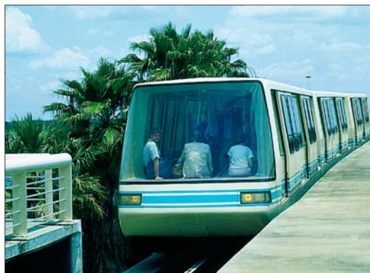
The People Mover monorail at Orlando International Airport
