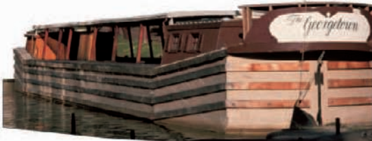
Passenger barge on the C & O Canal, a reminder of 19th-century shippers ㉑
