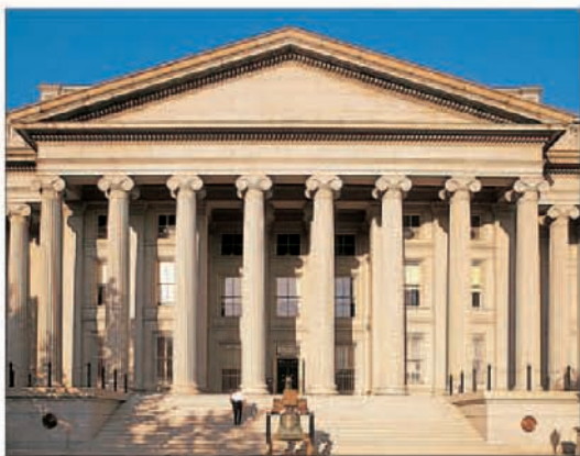
The colonnaded portico of the Neoclassical Treasury Building
