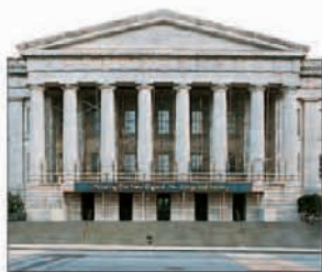
Façade of the building, housing the main entrance to both galleries
