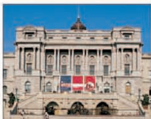
Front façade of the Jefferson Building
