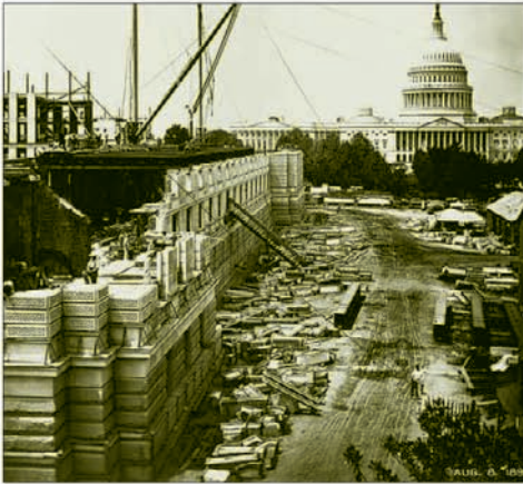
The Library of Congress under construction
