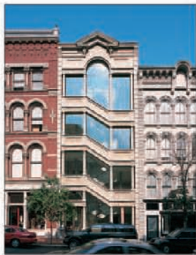
A contemporary office building linking two Victorian facades on 7th Street
