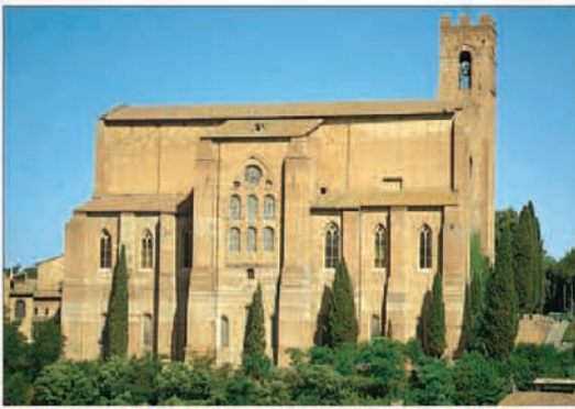
The façade of San Domenico
