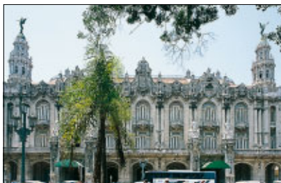
Façade of the former Centro Gallego building, now home to the Gran Teatro
