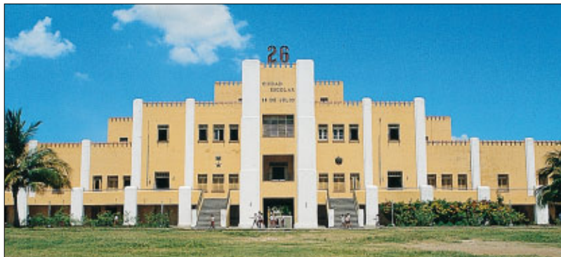
The impressive façade of the former Moncada army barracks, now a school and museum
