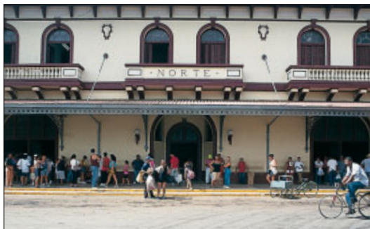
Façade of the railway station in Morón
