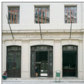
Entrance to a post office ( oficina de correo ) in Havana
