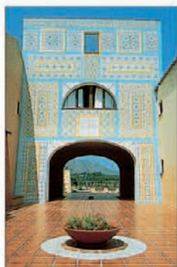
The Hotel Torre Moresca at Cala Ginepro, Orsei (see p175)
