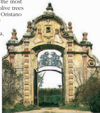
The 18th-century gate, Cantina Sociale
