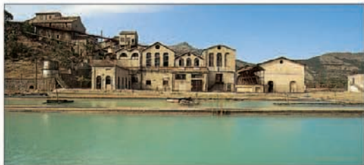
The large tanks at the Montevecchio mine
