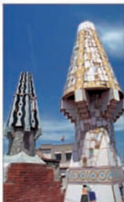
Palau Güell's spire-like roof chimneys
