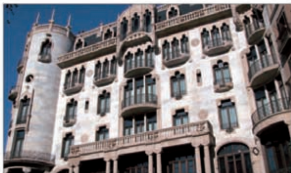
The façade of Casa Fuster, a Modernista building, now a hotel ③
