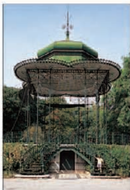
Attractive wrought-iron music pavilion in Jardim da Estrela
