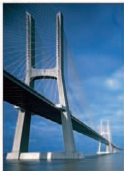
The vast Vasco da Gama bridge spanning the Tagus River
