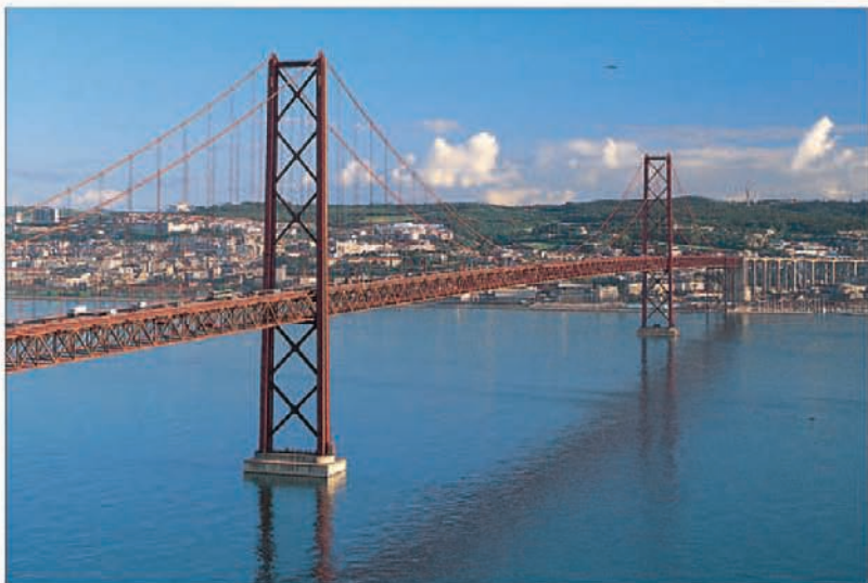
Ponte 25 de Abril linking central Lisbon with the Outra Banda , the south bank of the Tagus
