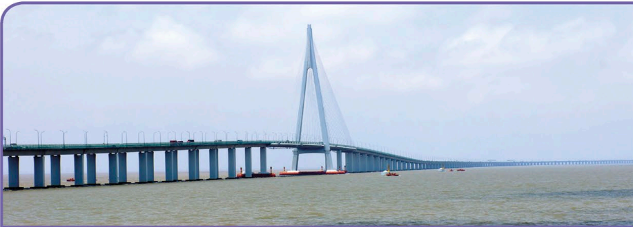
» Name: Danyang-Kunshan Great Bridge, China
