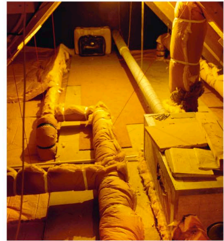
A heat recovery unit installed in a loft. The pipes running to and from the unit are lagged to prevent heat loss.
