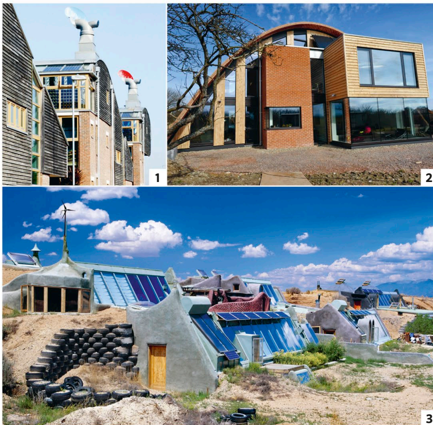
1. The first environmentally friendly housing development in the UK – Beddington Zero Energy Development (BedZED). Homes are made from reclaimed or natural materials. 2. A zero-carbon house in Kent, UK, needs no fossil fuels for heating. Its vault shape gives it high thermal mass. 3. Earth shelters in New Mexico, USA, are made from rammed earth and car tyres (see pages 48–49).
