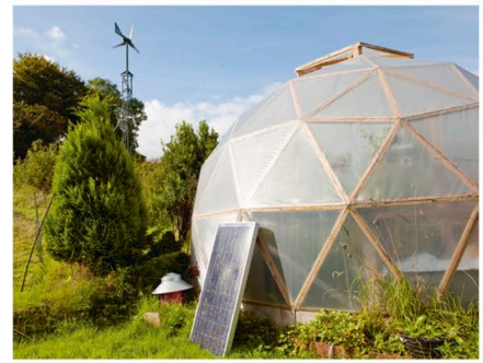
The shape of a geodesic dome avoids warm air pockets forming, making it ideal for growing plants under cover.
