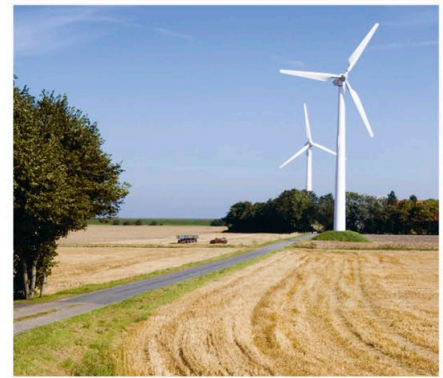
Flat farmland can be especially good for siting wind turbines as it has good laminar air flow.
