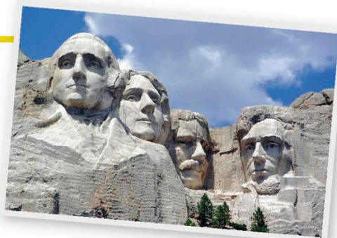
② Explosive dynamite was used to carve the four giant heads of these noteworthy American presidents into the rock.
