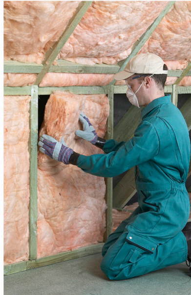
Insulating an attic
