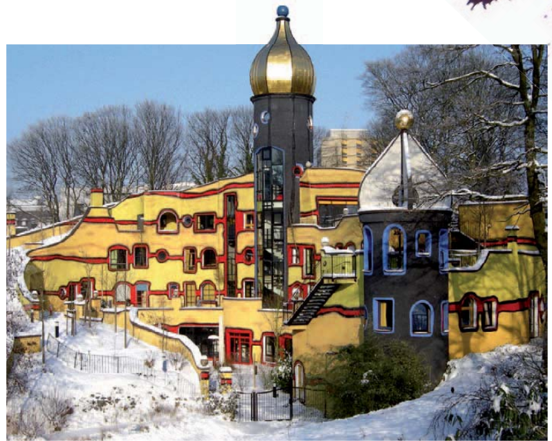
The Ronald McDonald House, Essen, Germany, completed in 2005
