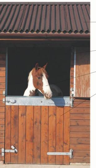
Roofing material must not be too noisy when hit by rain or hail, and must not become too hot in direct sunlight
