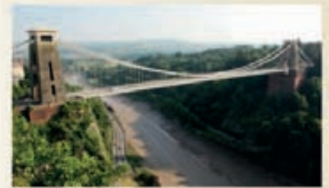
CLIFTON SUSPENSION BRIDGE, BRISTOL
