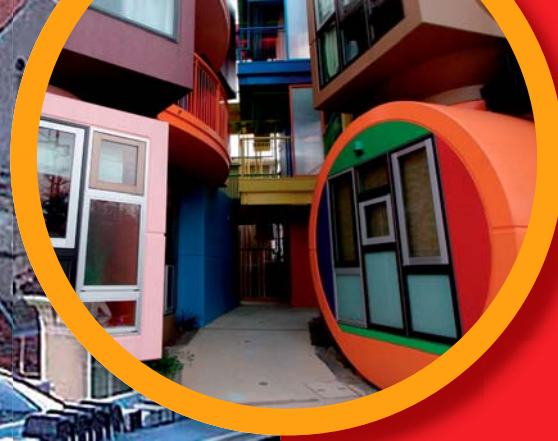
Tokyo technicolor This Japanese apartment building resembles a playground. While the exterior is a mix of colorful shapes, the fun continues inside with uneven floors!
