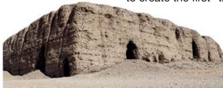
A mastaba was made of mud bricks. Inside, a deep chamber was dug, in which the dead were buried.
