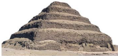
The Step Pyramid was designed as a stack of mastabas. It was made of small stone blocks laid like bricks.
