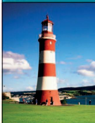
In 1756, John Smeaton built a stone lighthouse off the U.K. coast. He noted that unlike ordinary mortars of limestone and sand, those that also had a high proportion of clay became harder in water and could withstand the pounding of the waves. Shown here is the lighthouse, which was rebuilt on land as a memorial.
