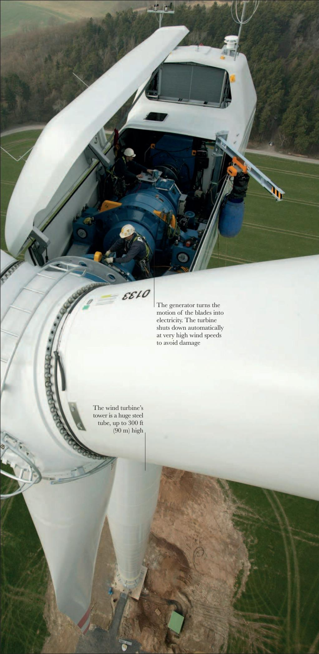
The generator turns the motion of the blades into electricity. The turbine shuts down automatically at very high wind speeds to avoid damage
