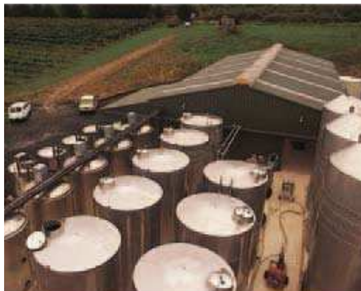
COOPERS CREEK WINERY, NORTH ISLAND
