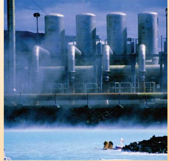
People in Iceland use the heat from volcanoes to make electricity. Pipes pump water through the hot rocks underground near a volcano. As the water heats up, it turns to steam. The steam is used to make electricity.
