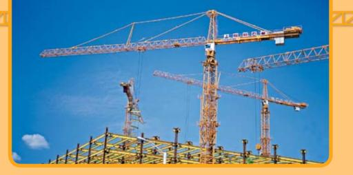
The **arm** on a crane can move up and down and left and right. The arm has big **blocks** at one end. The blocks keep the crane from tipping over as it lifts things.
